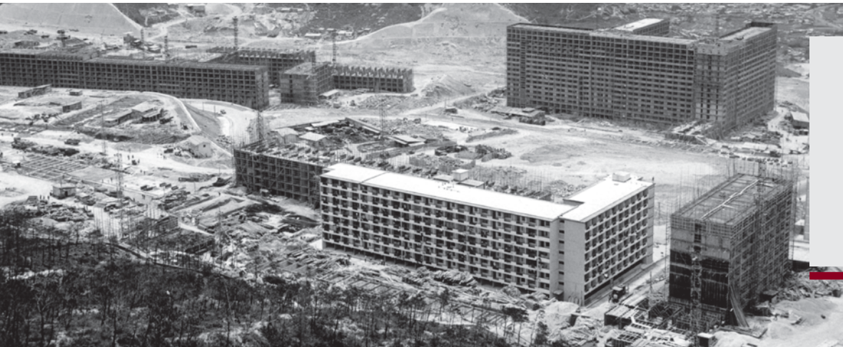
Tsz Wan Shan Estate (the term "resettlement" was gradually phased out) under construction. The completed building in the front is a Mark III block, while the unfinished structure behind, a 16-storey Mark IV block, 興建中的慈雲山新區（「徙置區」的稱謂當時漸漸不再使用）。前方已落成的大廈屬三型，後方興建中的大廈為樓高十六層的四型。（1965）
